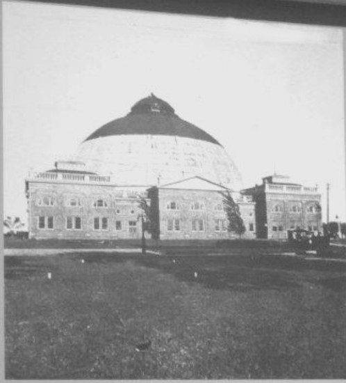
Dome Building - built in 1895
