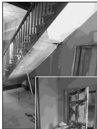
GETTING NEAR the refinishing line.
